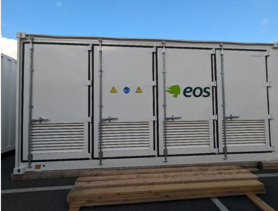
Frontal View of an EOS Zinc-powered Aqueous Battery Container
